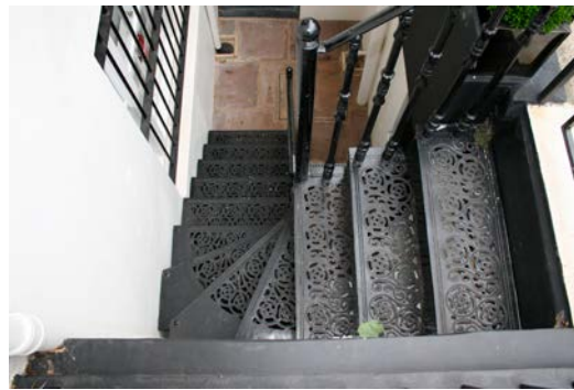
Victorian Kited Staircase
