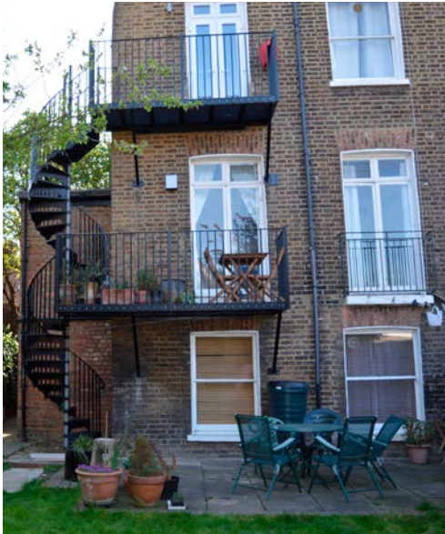
Double Flight LCC Spiral to Access Two Flats with Matching Balconies
